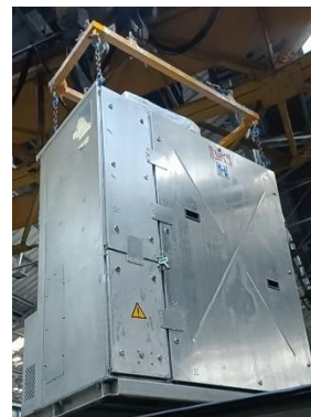
Fig 5.3: BOX2 Lifting arrangement
