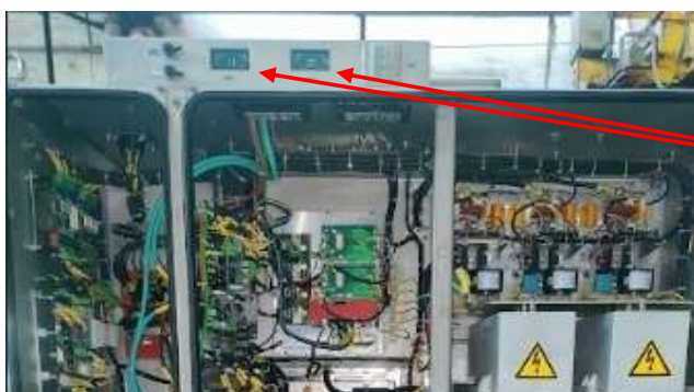
Figure 2- DC link voltage indicator BOX2 AUX1 & 2
