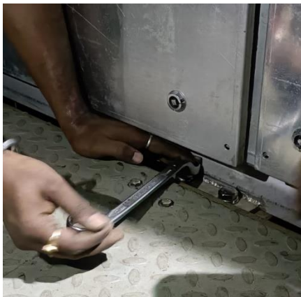
Fig 4.15.1: Base Mounting of Traction Converters
