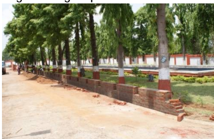
Construction work for the garden near C-D&D office campus
