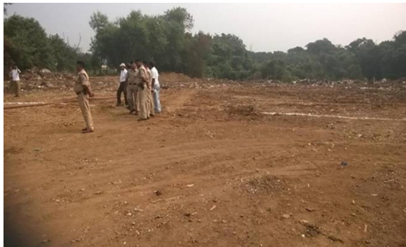
View after Cleanliness drive in shop premises
